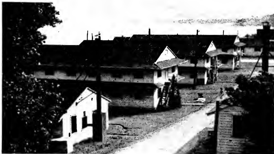
Army barracks at Fort Ontario, N. Y., remodeled to give each family its own apartment
